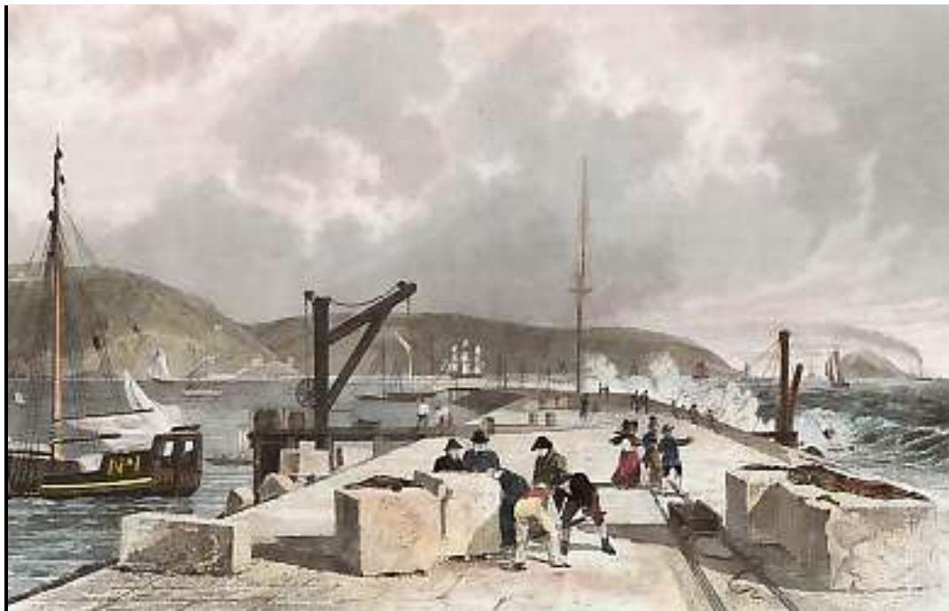
Breakwater looking from the West
