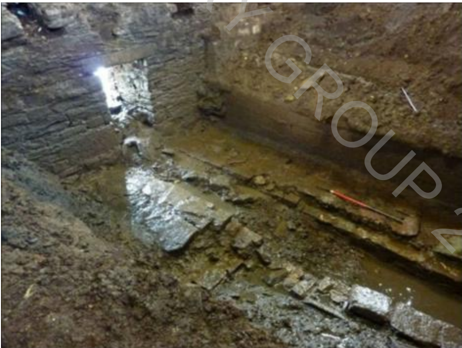
S4 Sluice channel and paved floor looking south east. Original granite quoins and lintel in the sluice opening. Joist holes from Phase 2 in wall above. Concrete blocking of sluice S3 beyond.
