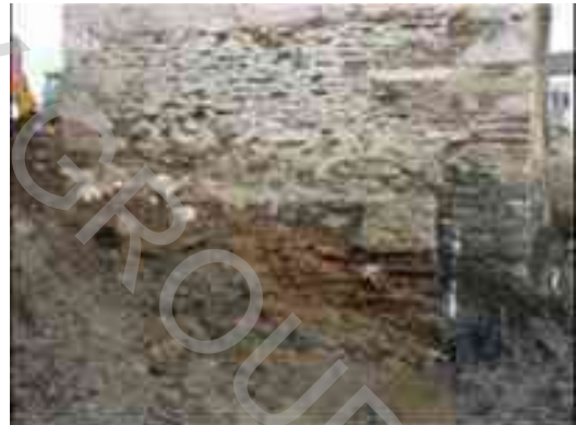
Stones re-used as quoins, St 7 to left, in south wall
