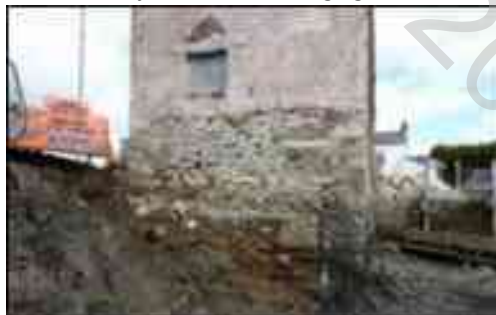
South face with remains of Mill Pool wall
