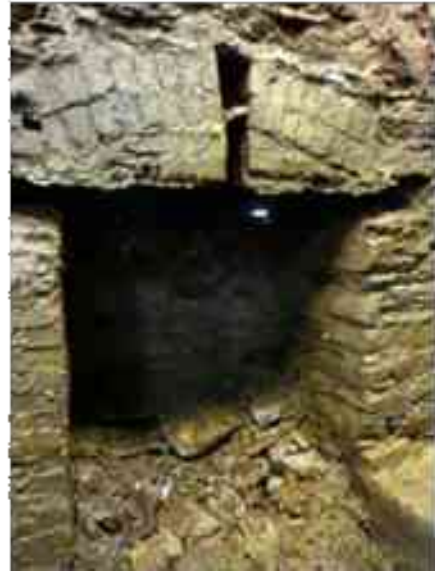
Detail of 19th century brick arch S5 in east wall
