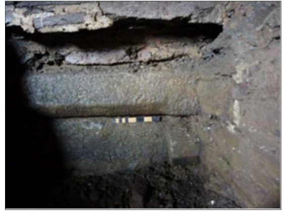
Detail of 16th century chamfered slab St 10 and mullion St 9 in the blocking of S3
