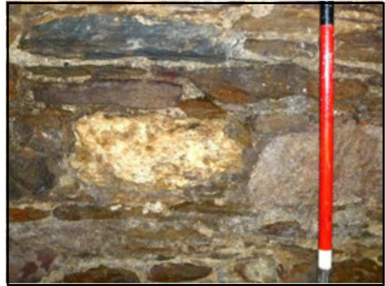
Fragment of French burr stone in north gable wall of mill
