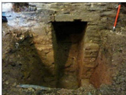
S4 west interior 16thC sill St 8 re-used as lintel
