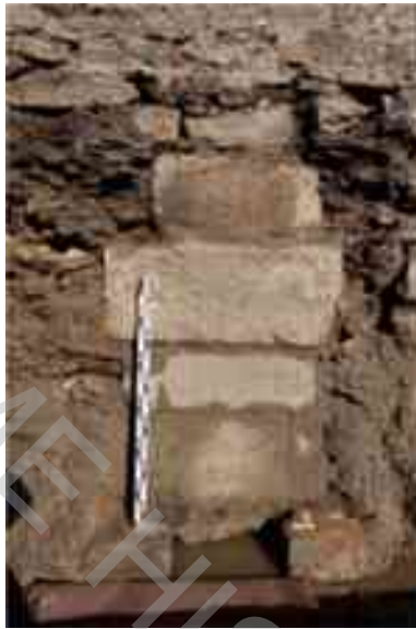
The granite blocking of Sluice 2. This small sluice which was probably part of the 16th century mill has rather less elaborate sluice board stones at the base but no lintel over the blocking
