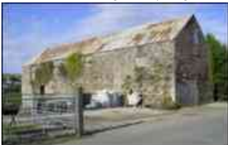
East and north faces showing Extension
