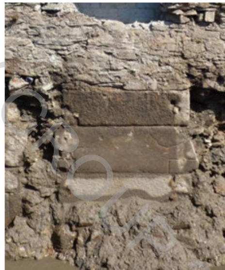
The granite blocking of 19th century sluice S5: this blocking is also made up of granite slabs which may have been capping stones
