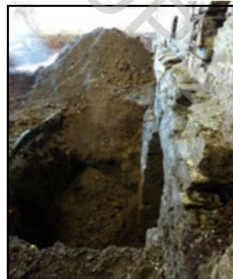
View along the west wall a looking south. Showing Offset B above Offset A which is assumed to be the top of the 16th century build. The Phase 2 mill was slightly re-aligned above Offset B.
