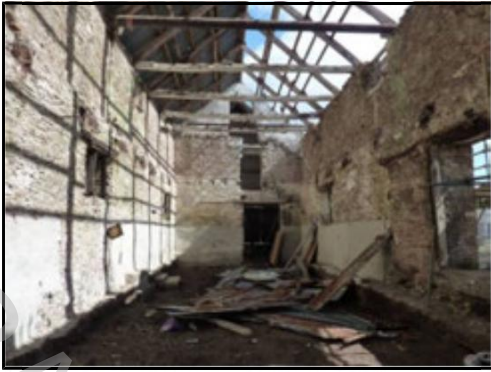
Looking north with roof being removed
