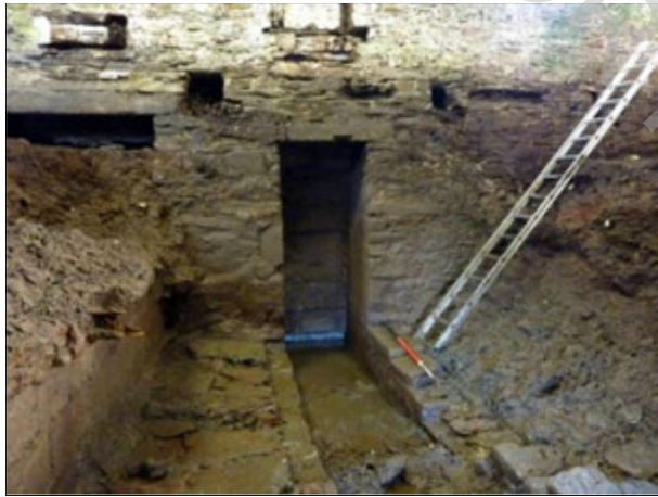
Basement: West wall with sluice S3 and concrete blocking to left. Sluice S4 with granite lined water channel and paved floor, granite quoins up to Offset A. Phase 2 rebuild above with re-used 16th century lintel, joist holes below Offset B and blocked sluice control features F1 and F2 above
