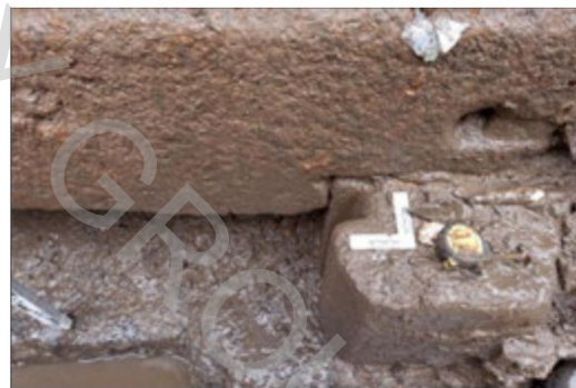
Details of Sluice S3: seating for sluice boards possibly 16th century
