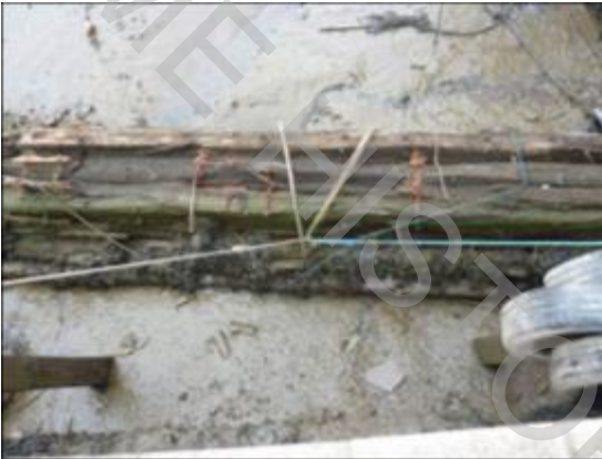
Pontoon showing iron bolts and spikes
