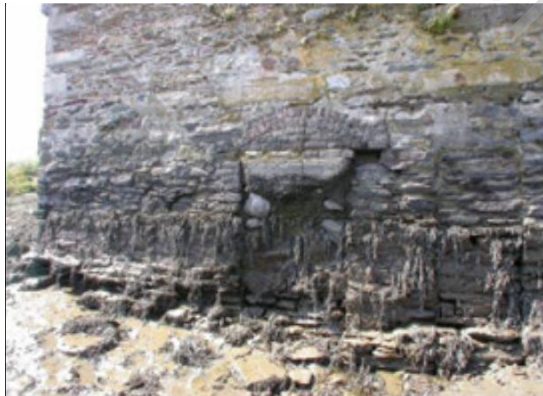
Details of the sluice arches in the east wall: left S1, S5 and S2. Right S3 and S5
