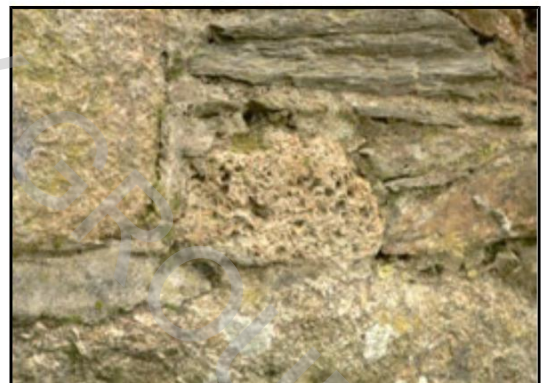
Fragment of French burr stone built into east wall of mill
