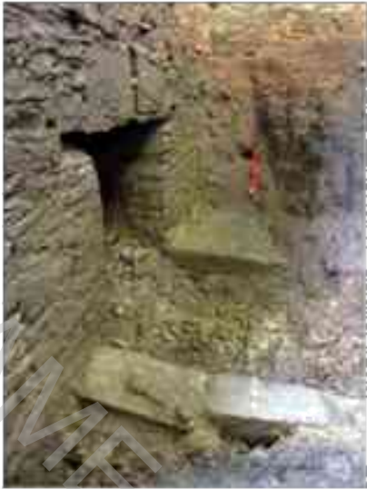
Sluice S5 granite edging of water channel
