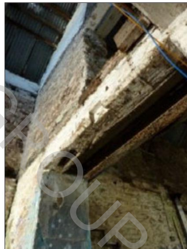
Looking up to wooden lintel and steel joist of door D3
