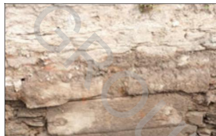
S3 west exterior 16thC sill re-used as lintel
