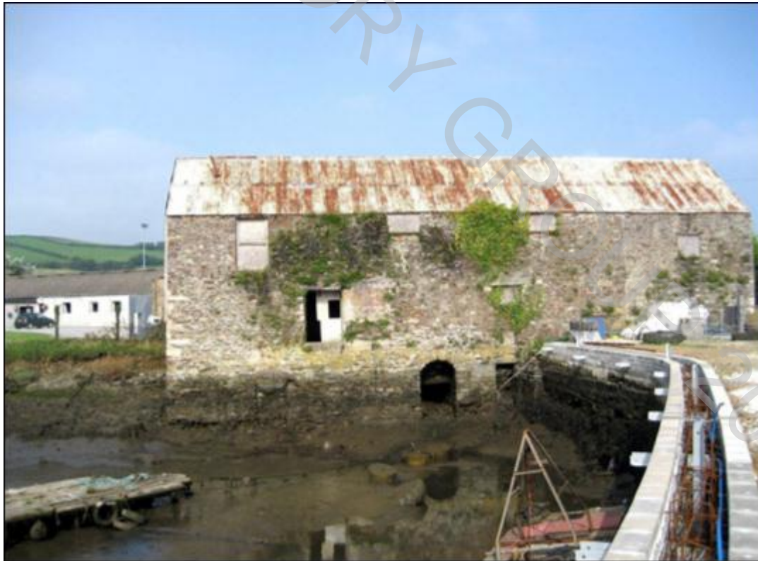
East Wall in 2008 showing the Football club building to the left
