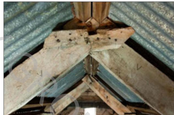
Looking south: apex truss V
