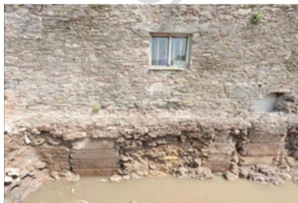
West wall face, blocked sluices, left to right- S3, S2, S5.
