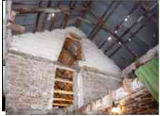
Area A Looking south up to doors D5 (above) and D4 (below). D5 was the original opening in the north wall of the main mill for hoisting sacks into the loft; D4 was broken through when the Extension was added
