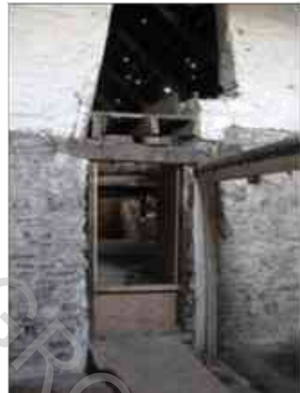
Area A Looking south up to doors D5 (above) and D4 (below). D5 was the original opening in the north wall of the main mill for hoisting sacks into the loft; D4 was broken through when the Extension was added
