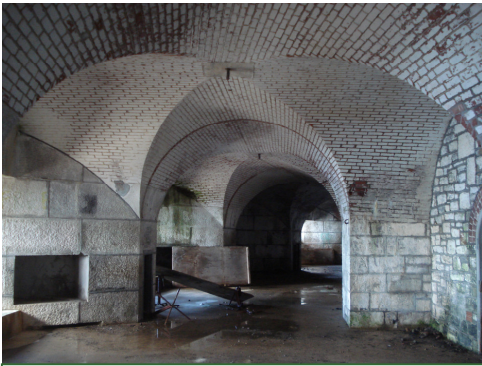
The interior of the garden battery today
