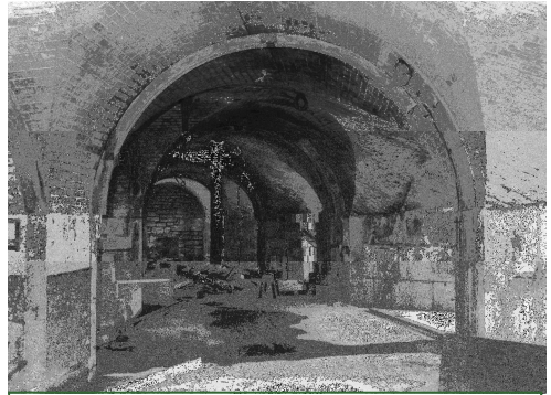
Picklecombe interior before conversion (1970s)
